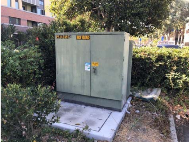
7. View of the subject property pad-mounted transformer
