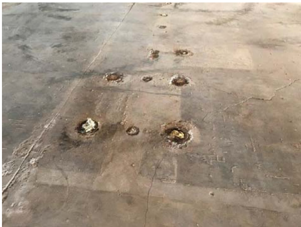
15. View of the subject property previous use floor mounts and cutouts
