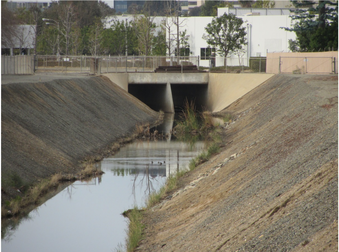
Photo 2 - View of Barranca Channel at the entrance to the RCB under the AT&SF Railroad Spur. This RCB is located upstream of the proposed Kelvin Pedestrian Bridge location. (Approximate capacity of 750 cfs.) Note restriction of existing box culvert at Barranca Channel.
