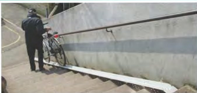
Figure 3.1 A bike trough located along a staircase can allow for safe, continuous active transportation through the intersection
