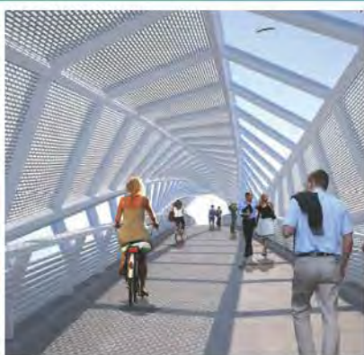
Figure 2.9 TYLI recently designed the Hillsdale Pedestrian Bridge in San Mateo, CA, which utilizes a weave truss to create a unique user experience similar to what could be applied to the Jamboree/Michelson Pedestrian Bridge.
